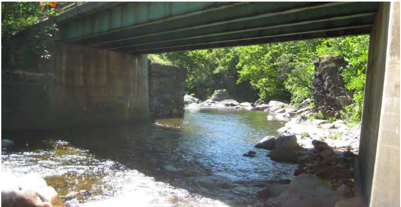
Figure 8. - Looking at bridge from upstream. Left Abutment is at left of photo. Note flow against Left Abutment. Right abutment is on bedrock.
