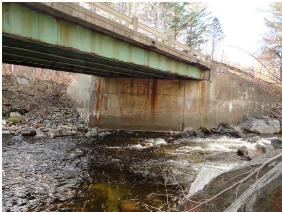
Figure 6. Phillips - Looking at Right Abutment center), note old stone abutment (left in image). Upstream is on right of photo
