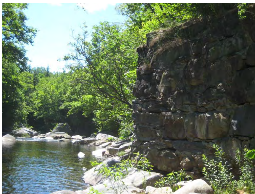
Figure 12. Looking Downstream from Bridge. Note old abutment on right. Old abutment set on rock.
