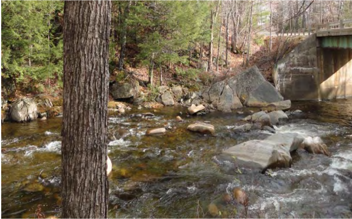
Figure 7. - Looking at Bridge from upstream. Looking at Left Abutment. Note projecting rocks into Left Channel.
