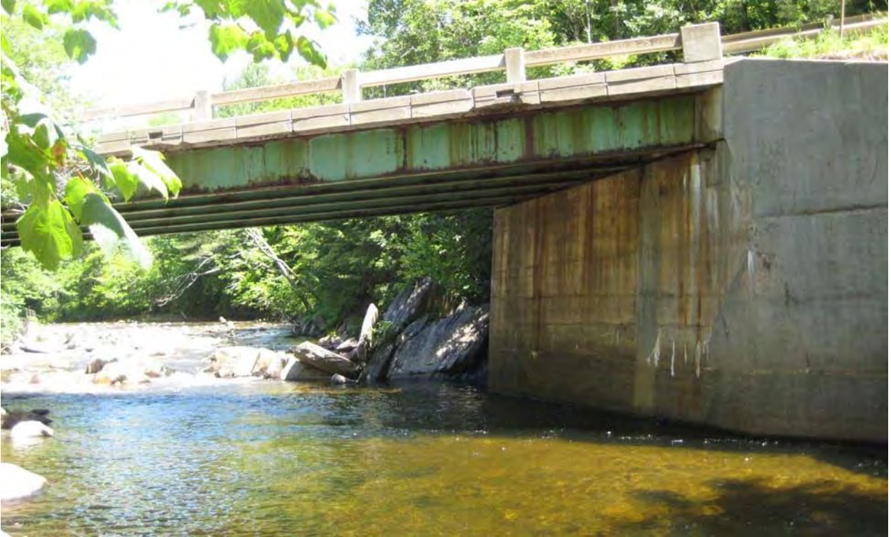
Figure 13. Left Abutment. Note deep flow against Abutment, and rock projecting just upstream of the bridge.
