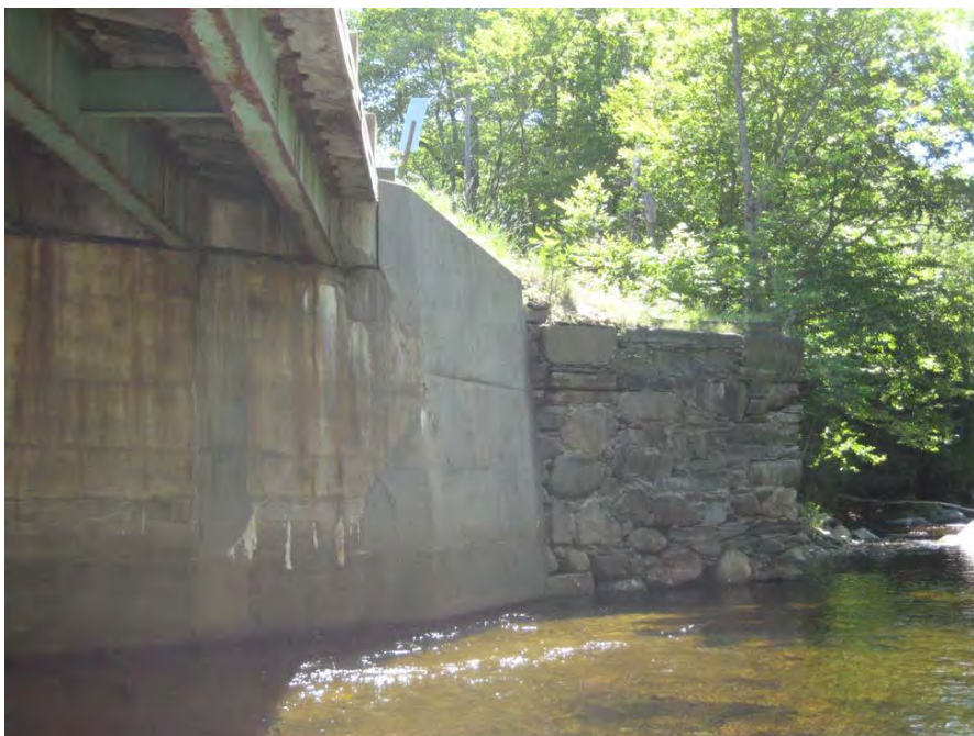
Figure 11. Looking at Left Abutment. Note old rock abutment downstream of existing bridge.
