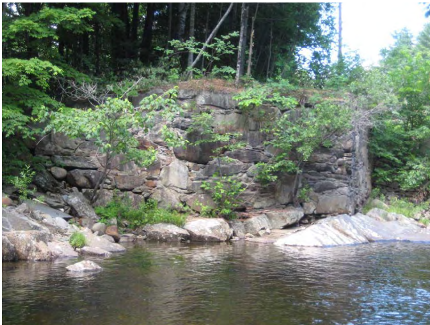
Figure 14. Abutment for former bridge on Right bank, downstream of existing Bridge
